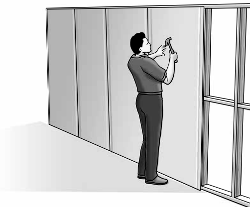
Figure 4: Fixing remaining sheets
